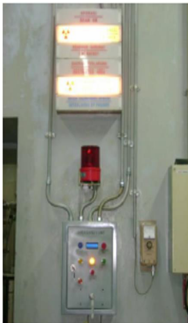
(a) The cave control unit is at the front of each cave (b) Area radiation monitor for all caves Fig. 2. (a) Cave control unit located at the front of each cave (b) Area radiation monitor for all caves
