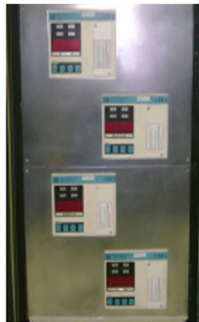
(a) The cave control unit is at the front of each cave (b) Area radiation monitor for all caves Fig. 2. (a) Cave control unit located at the front of each cave (b) Area radiation monitor for all caves
