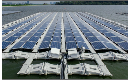
Fig. 2. Pontoon based floating PV system [14]
