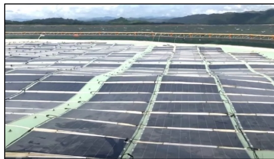
Fig. 3. Flexible floating PV system [15]
